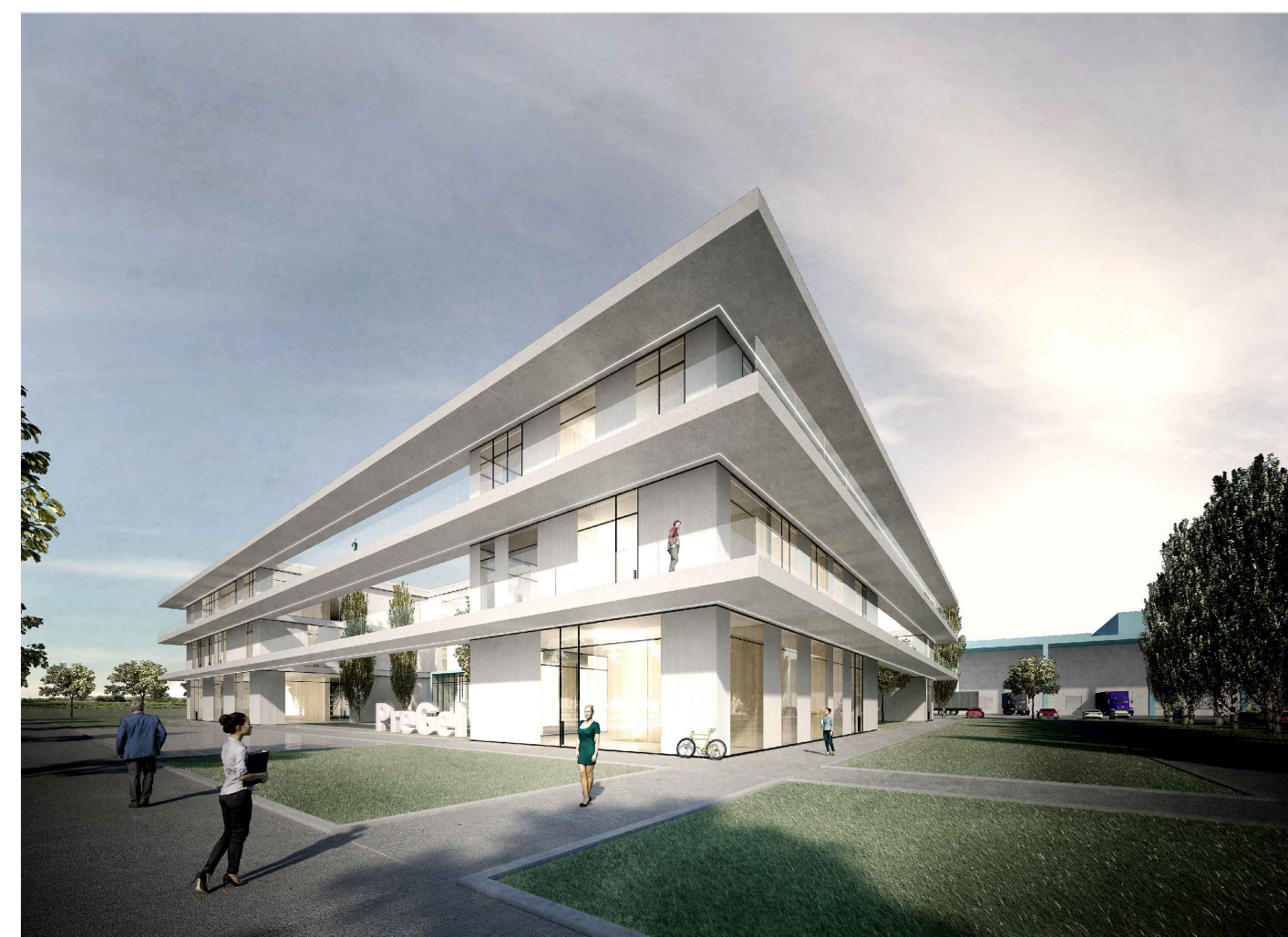
01 - HEADQUARTER - VISTA ESTERNA
